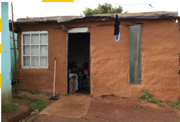
Figure 1: backyard-bedroom studios, exterior view
